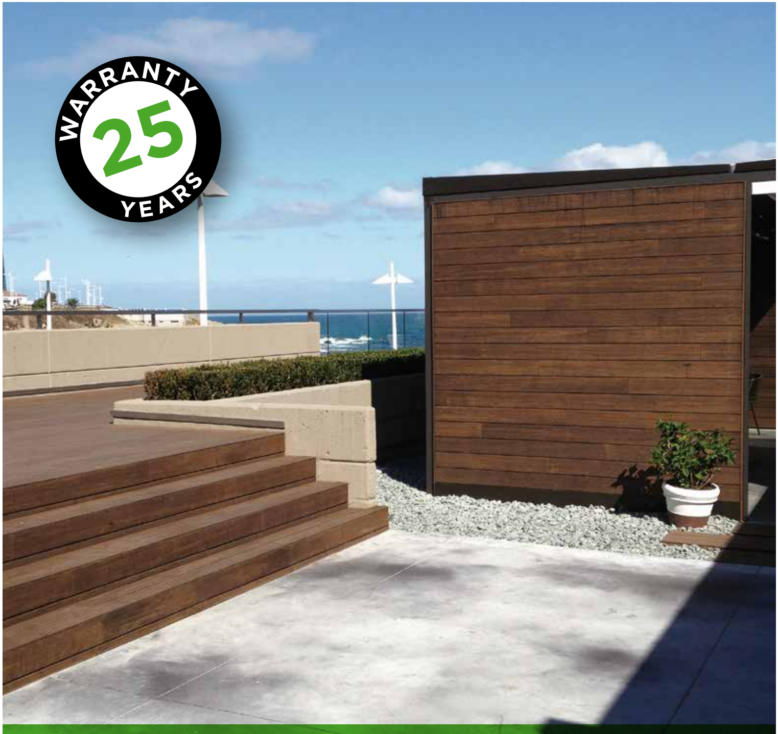
MOOM 57 Restaurant (400 m 2 ) La Coruña, Spain
