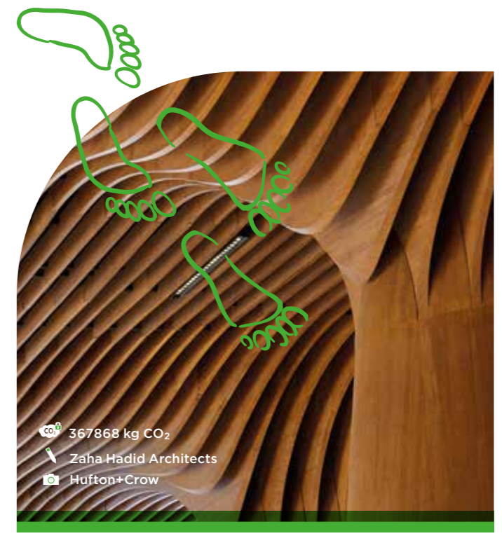
CityLife Shopping District - Podium Zaha Hadid LEED Gold - (10,000 m² + 70,000 m²) Milan, Italy
